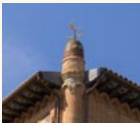
Cylindrical cap crowning the building.
